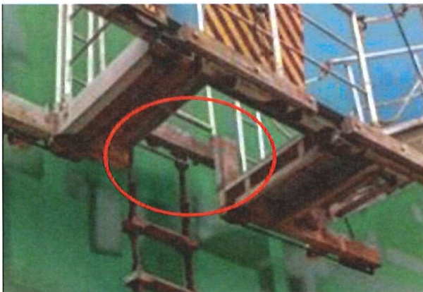
Figure 1: Pilot ladder/trapdoor showing the non-compliant horizontal cross-member.
